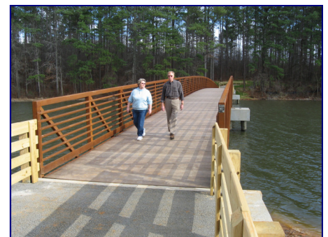
Acworth residents Red and Shirley Walker walk across the new bridge that links Cauble Park to Winn Street.
